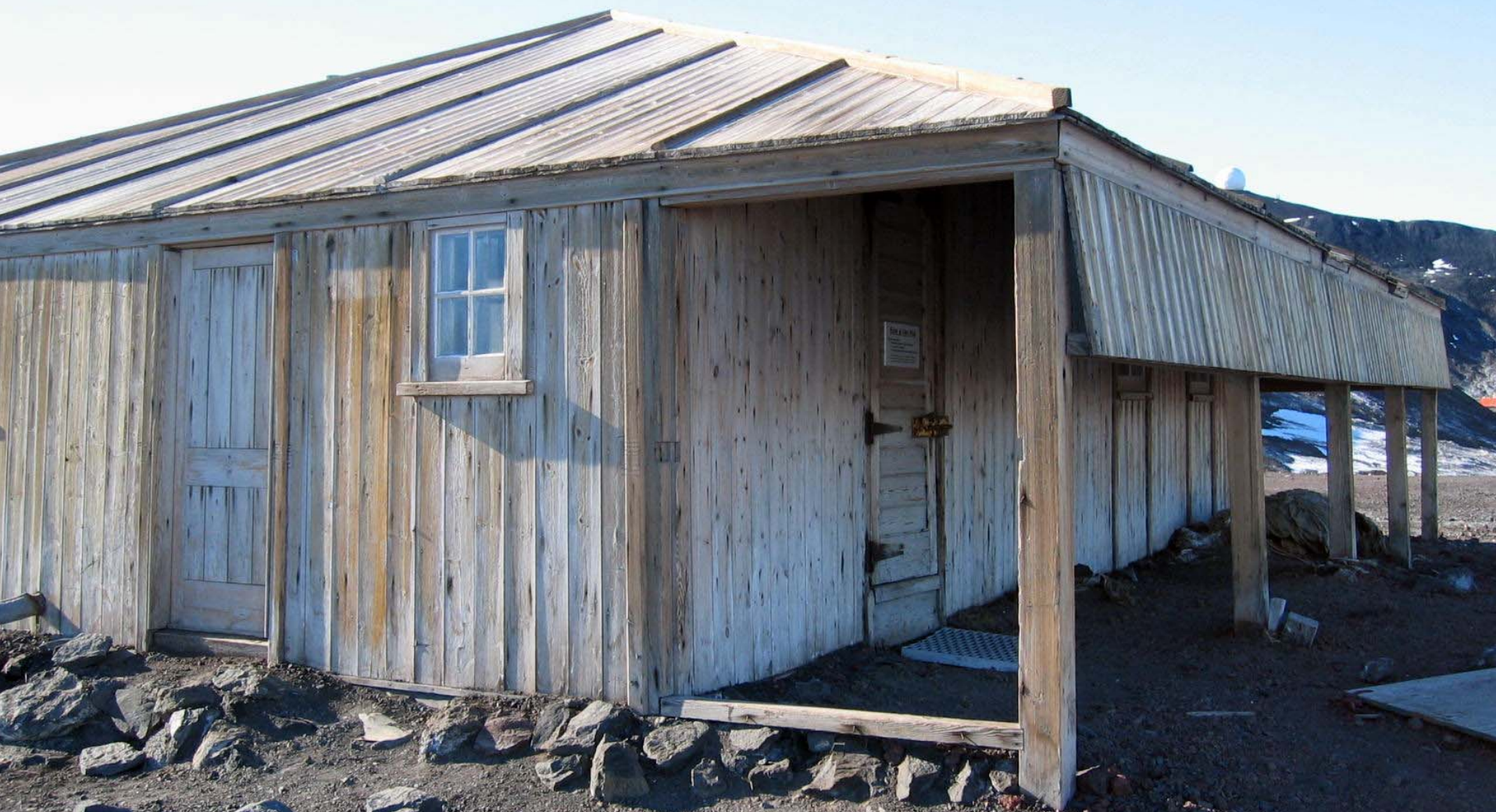
COMMANDER SCOTT'S 'DISCOVERY' HUT, HUT POINT
