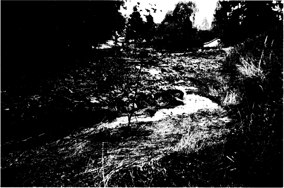
Fig. 3. Photograph of the floodplain below Reservoir No. 3, Centralia, Wash., where there was only minimal damage from the flood.
