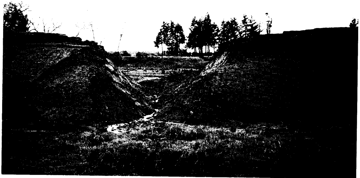
Fig. 5. Photograph of breach and slump failure of the Porter Hill dam, near Roseburg, Oregon.
